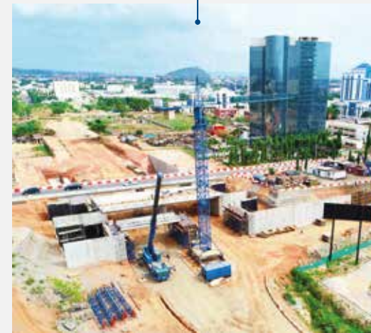
Central Roads, Abuja
