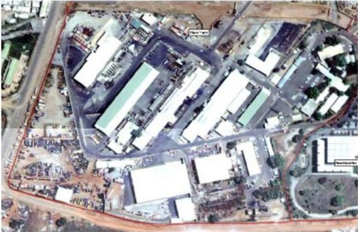
Figure 3: Main Yard, Abuja
