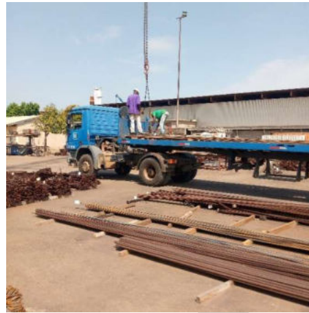
Figure 1: Tagged Reinforcement steel supplied to site from AID Figure 2: Storage of reinforcement off the ground
