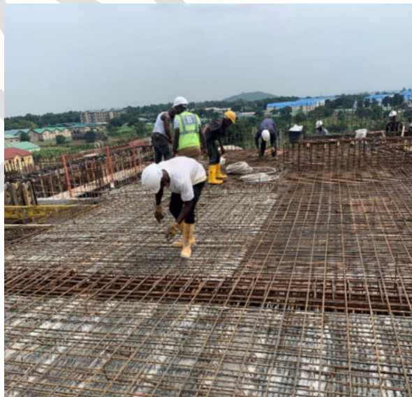
Figure 3: Reinforcement Fixing and Placing
