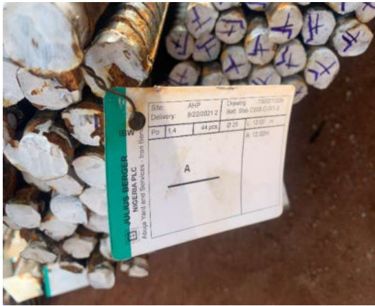
Figure 1: Tagged Reinforcement steel supplied to site from AID Figure 2: Storage of reinforcement off the ground
