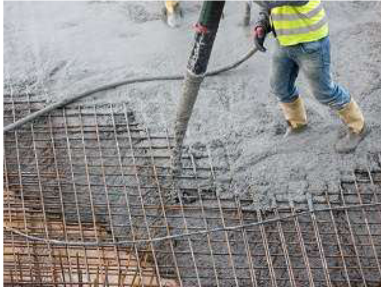
Figure 4: Pouring of Concrete
